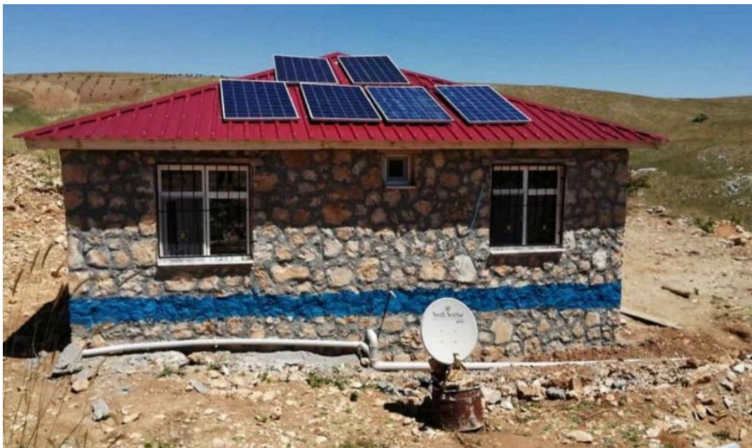
Photo: Stone House, Solar Panels
